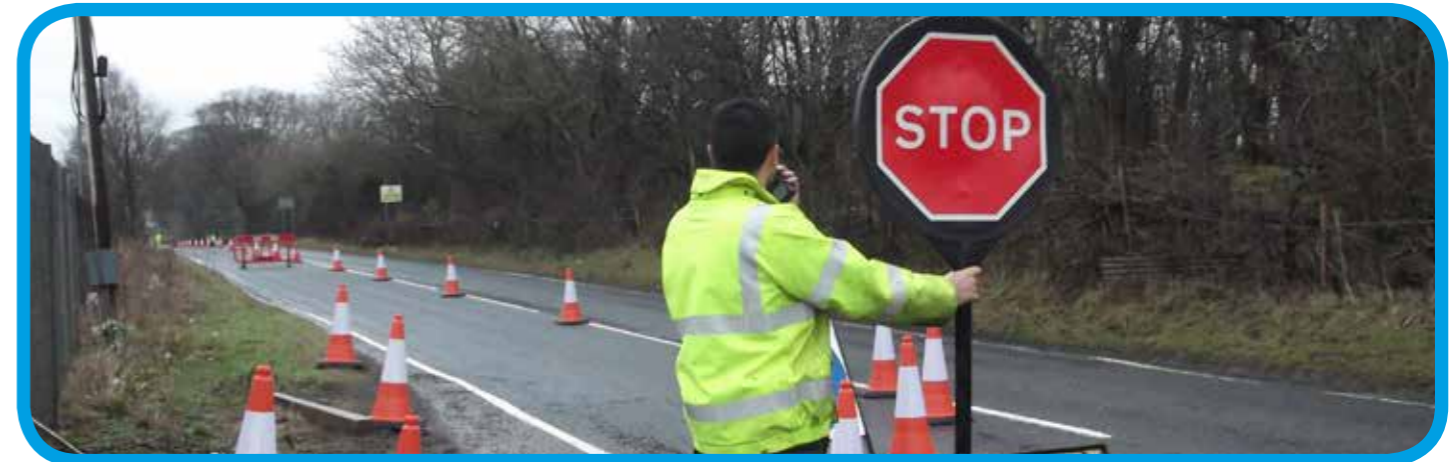
Defect and Priority Table 7:
